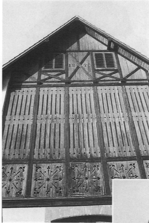
Abb. 9: Grenzach, Schlöble-Scheune, 1873 (Foto: H. Bauckner)
